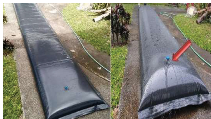
Figure 6. Filling of rectangular pillow tank (left); Pressure valve releasing excess water from the tank (right)
