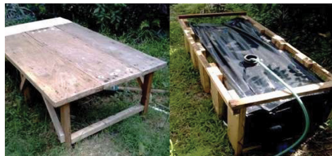
Figure 11. A wooden stand is an optional feature to elevate and secure the tank
